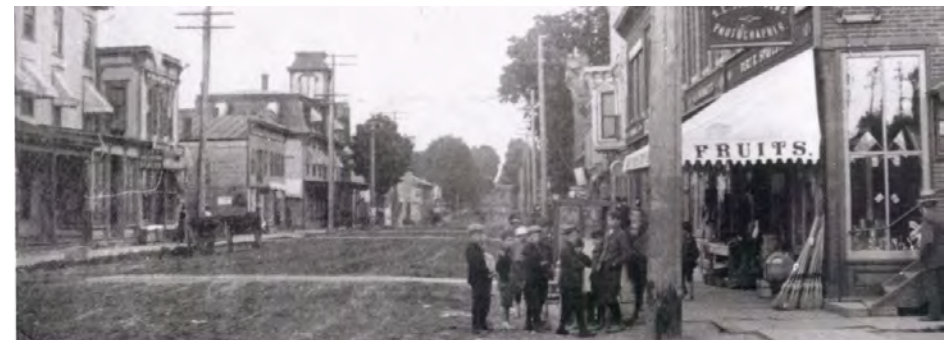
Figure2 Building located at 5 East Main Street
